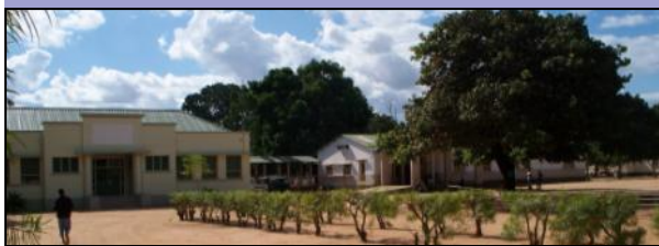
The entrance to the Rural Hospital of Montepuez.
