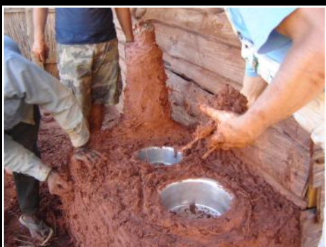
Jeremy, Kyle and Rusty build a Lorena stove
