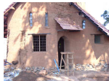
A recently completed cob structure at our property
