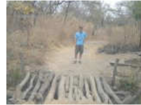
Chad inspects one of the bridges on the road to Lichinga
