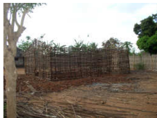
Construction of a church building in Nanhupo
